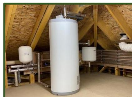
PLANT INCLUDING THE CYLINDER INSTALLED IN THE LOFT SPACE
